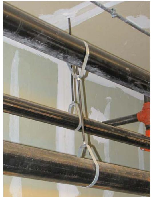
This pipe should be suspended from the structure, not another pipe.
